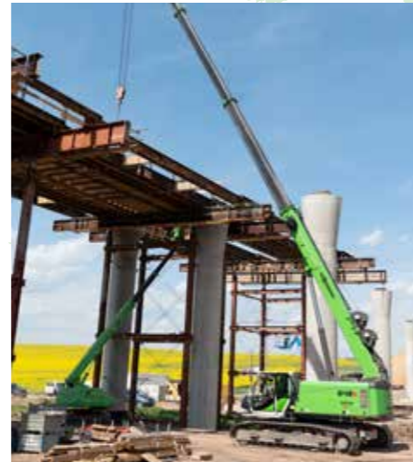
Bridge building Brückenbau
