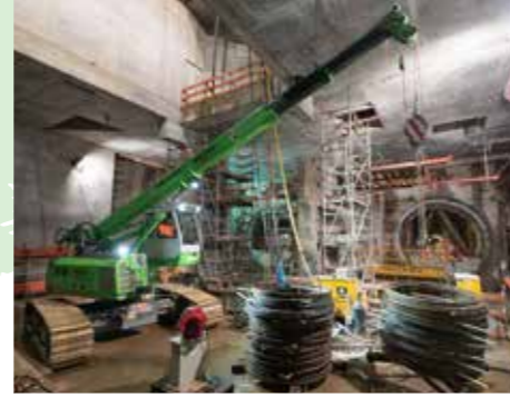
Tunnel construction Tunnelbau
