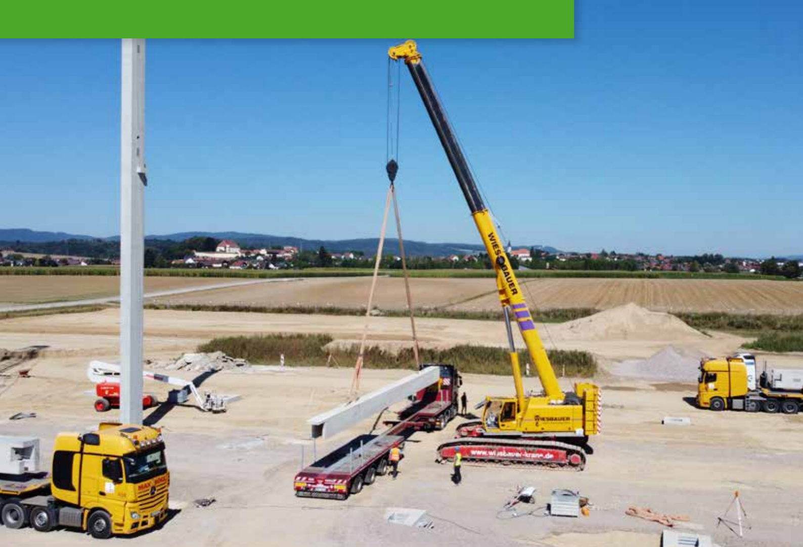
6113 R - Unloading heavy parts from trucks in pick and carry operation; Germany 6113 R - Entladen schwerer Betonelemente im Pick and Carry Einsatz; Deutschland
