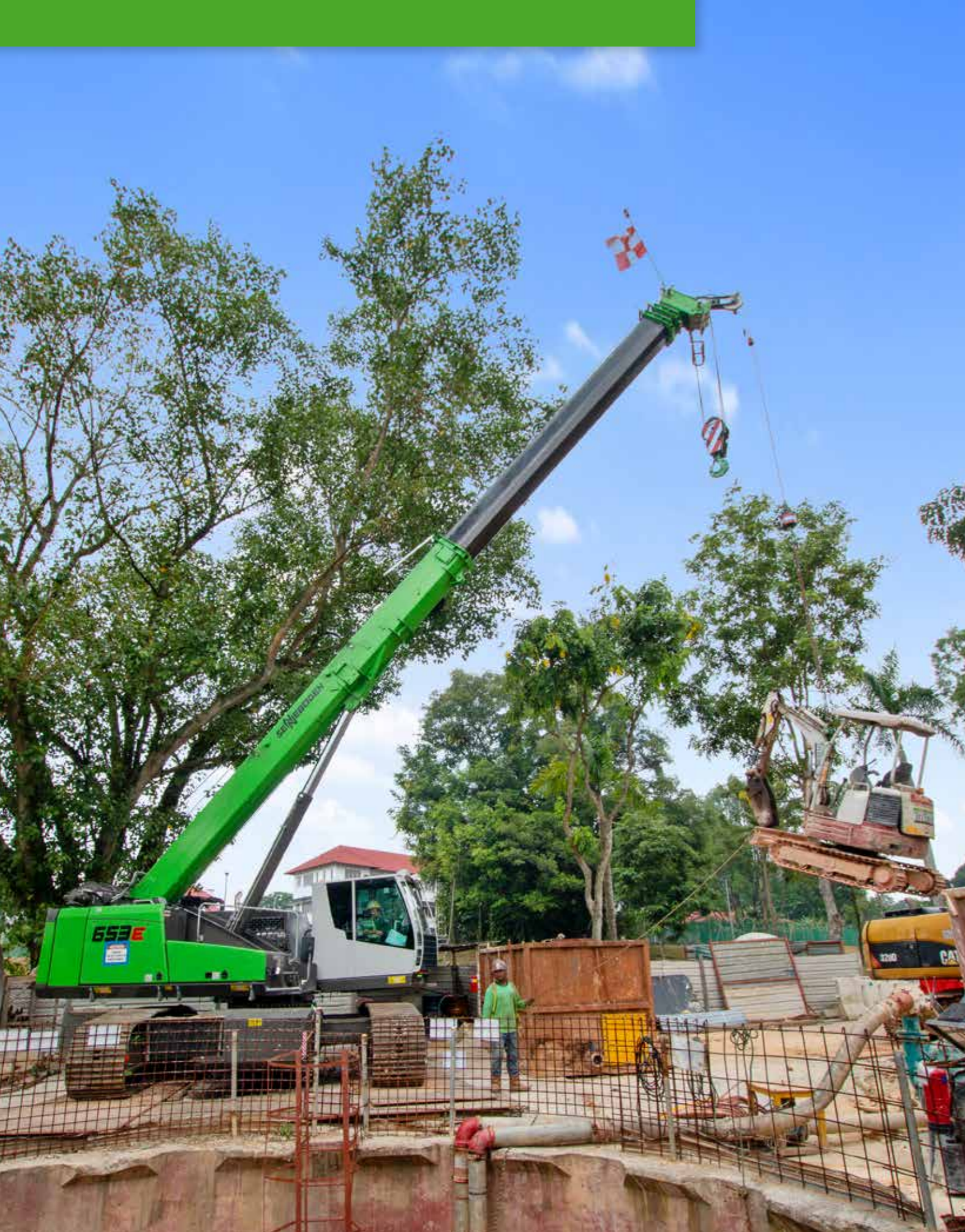
653 R - sewer construction; Singapore 653 R - Kanalbau; Singapur
