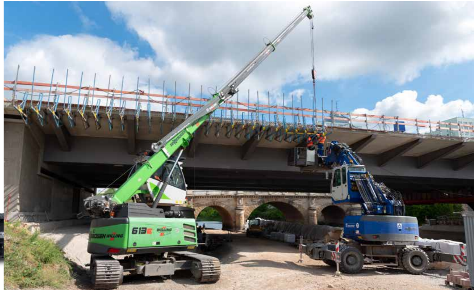
613 R - bridge building; Germany 613 R - Brückenbau; Deutschland
