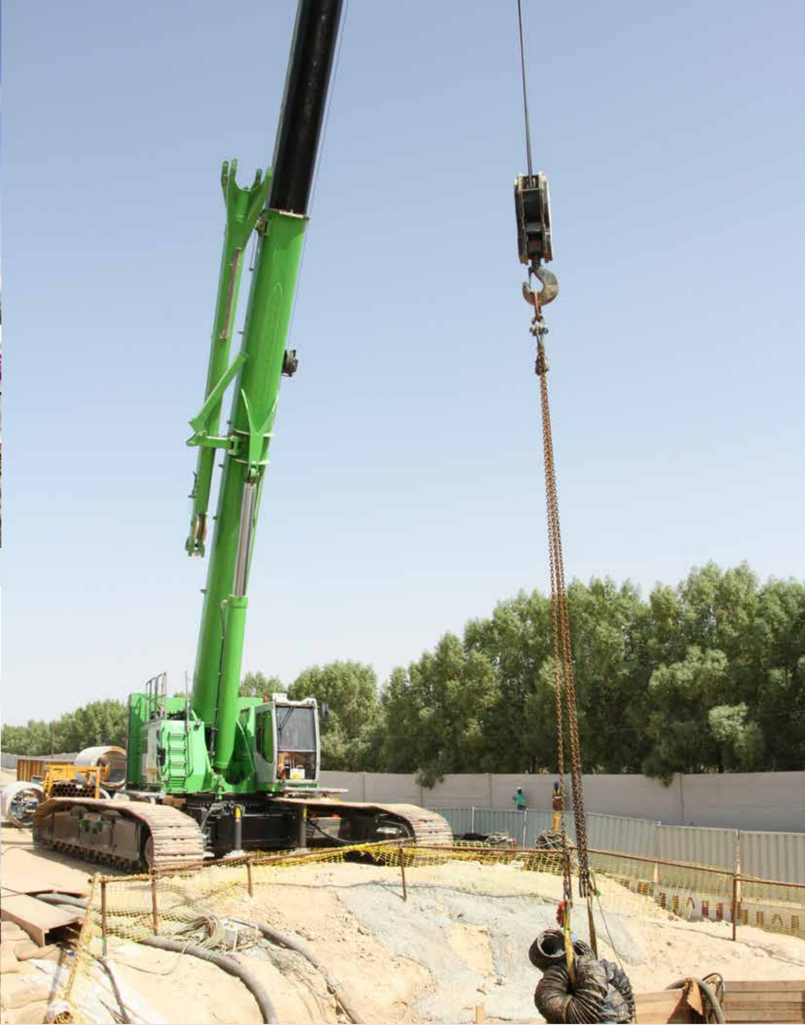
6113 R - Microtunneling; Dubai 6113 R - Microtunneling; Dubai
