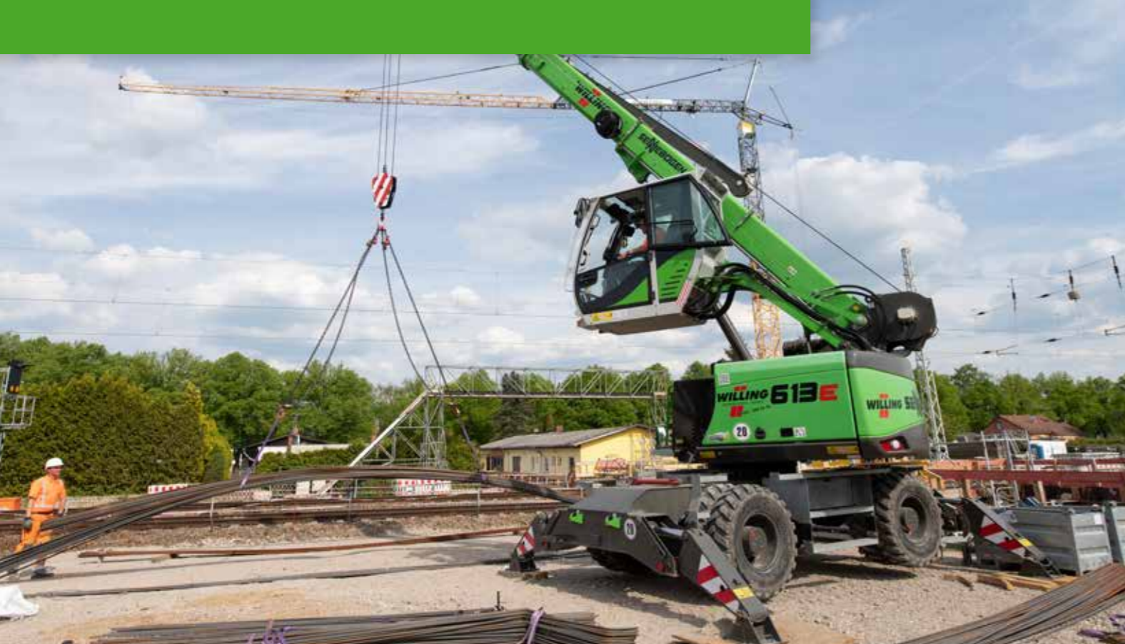
613 M – suburban railway construction; Germany 613 M – S-Bahn-Bau; Deutschland
